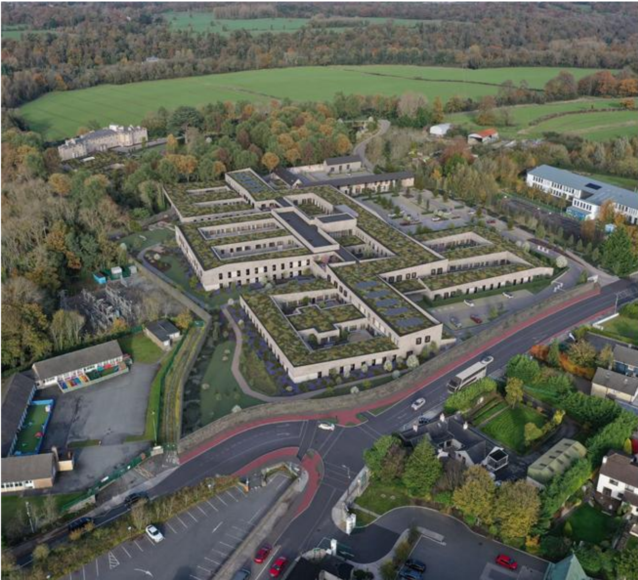
Figure 1-3: Aerial View of the Proposed Development
